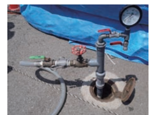
Injecting microorganisms into soil to break down chlorinated ethylenes
