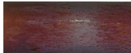
Iron compounds in supply water are attached to the heat-transfer surface of a test tube
